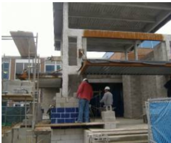
Gymnasium Front Entrance
